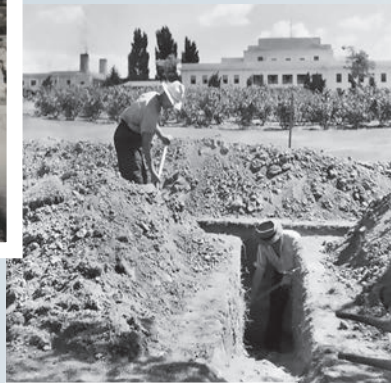
Old Parliament House, 1940s Workers digging slit trenches on the land of the old Parliament, in preparation for an air raid. The Canberra City Band playing at the ANZAC Day Ceremony at the War Memorial, 25 April 1948 www.aem.gov.au
