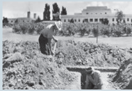
• Workmen digging trenches in preparation for an air raid, Canberra, Australia
